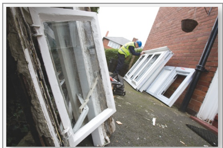
Low maintenance recycled PVC windows replace timber frames
